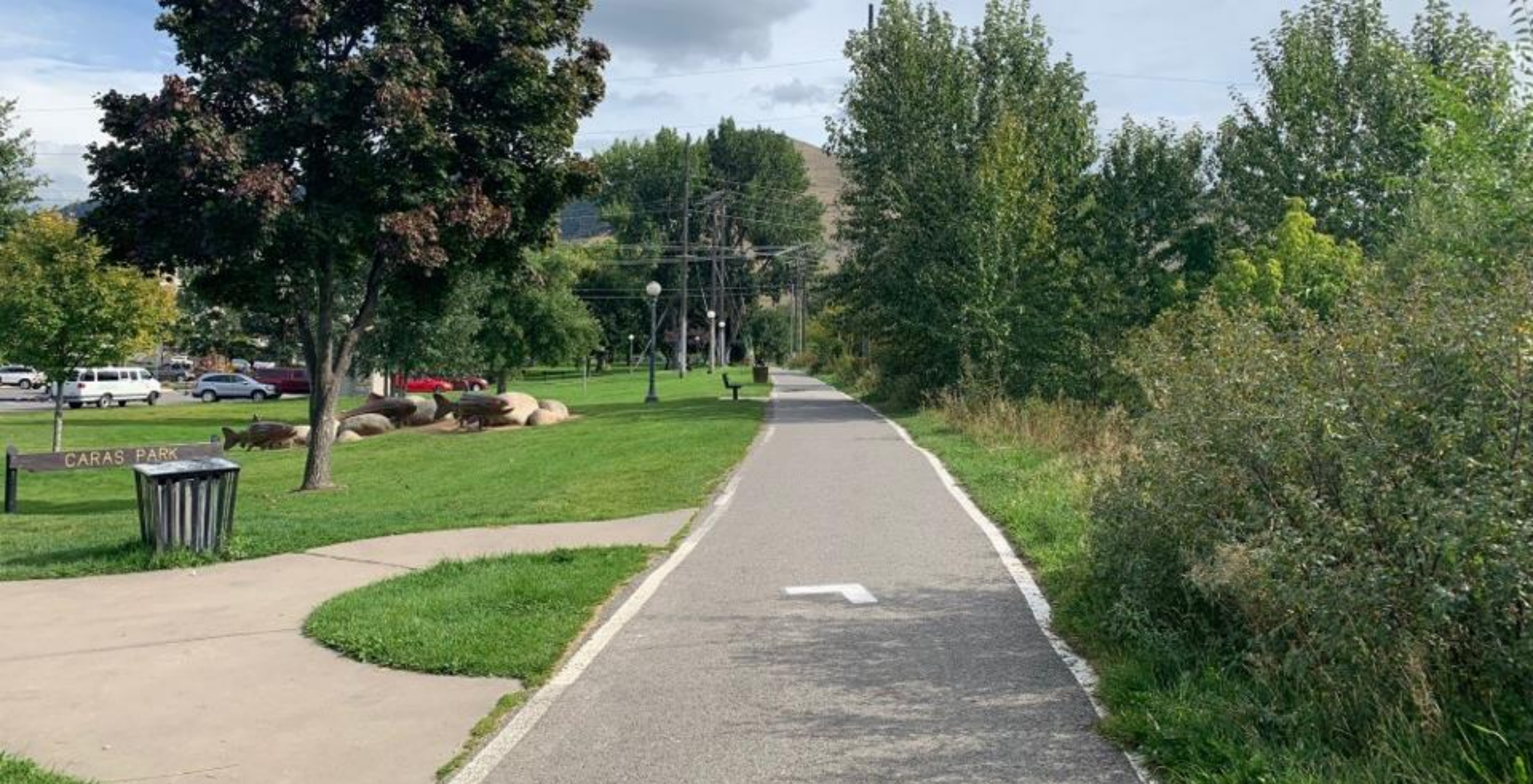
EXISTING SHARED USE PATH ALONG RIVER
